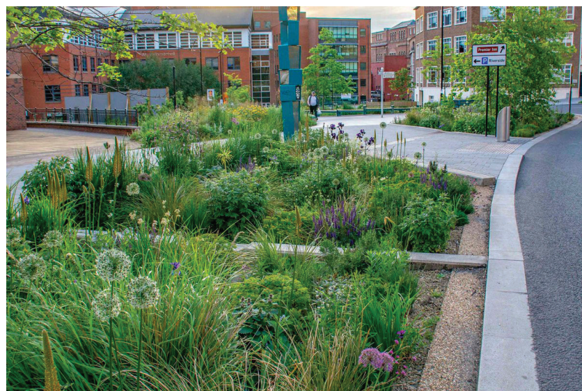
Fig. 4.29.6: Example of Sustainable Drainage Systems (SuDS)
