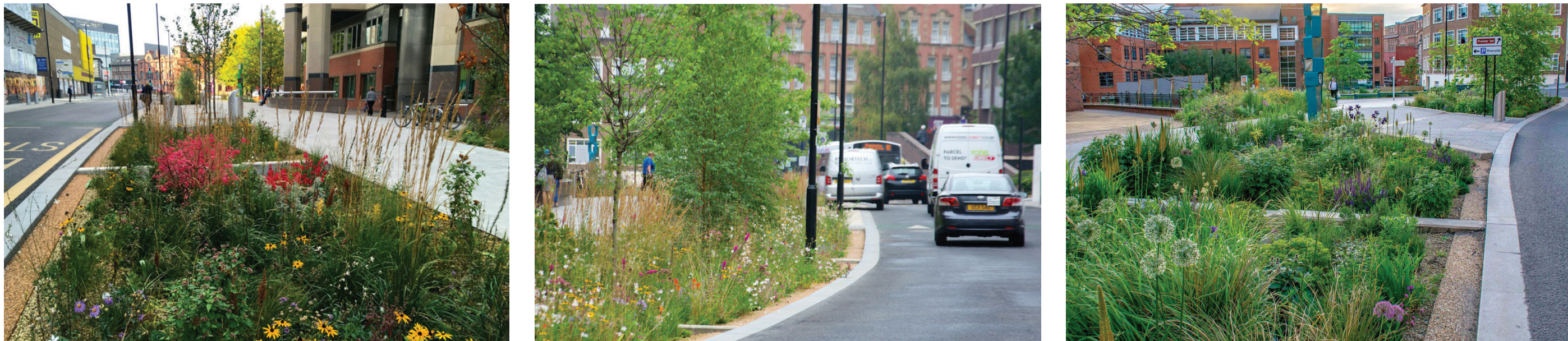
Fig. 4.29.10: Images of Planted Swales (Sheffield Town Centre)
