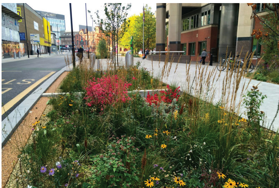
Fig. 4.29.3: Example of Sustainable Drainage Systems (SuDS)
